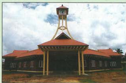
New building of Agricultural Technology Information Centre
