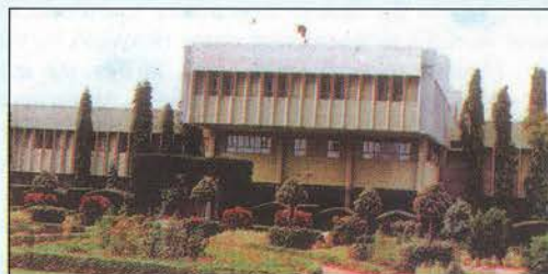
University Administration Building
