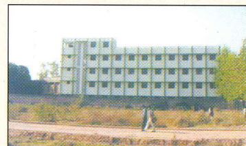
A Section of new built girl's Hostel
