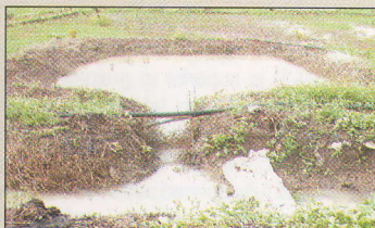
Percolation pit-cum-bore well to harvest rain water
